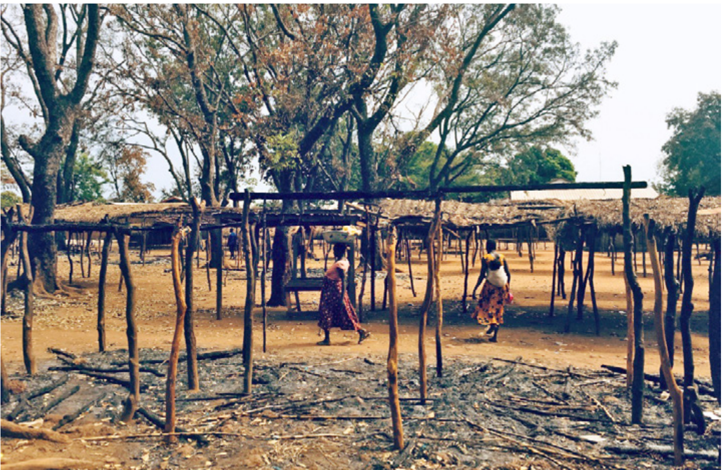
PICTURE 4. Burnt central market, November 1 st 2018.
